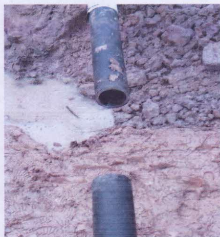
Fig E&F: Incident facility during repair
